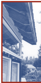
Open eaves, vents not screened (6 pts)
