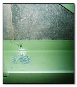
Light green paint on the interior steel ceiling trusses and asbestoscontaining grey panelling (Sample 17A-AREB-15) covering the interior ceiling of the AREB.
