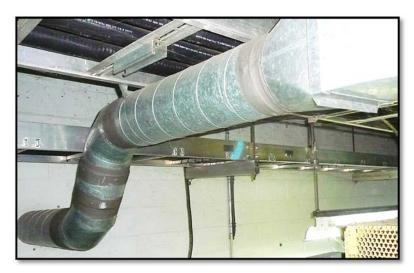
Sample 17A-AREB-04A - grey mastic on supply ducting was 'None Detect' for asbestos.
