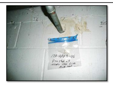
Sample 17A-AREB-06 - fire stop at the gas line on the northeast wall of the AREB was 'none Detected' for asbestos.
