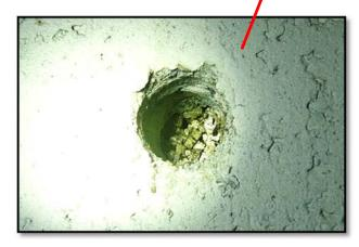
The vermiculite insulation as observed within the concrete masonry unit (CMU) walls of the 480 Volt AEB is assumed to contain asbestos and by WorkSafeBC criteria is classified as an asbestos-containing material.
