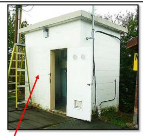
The smaller older eastward 480 Volt Aeration Electrical Building (AEB). The concrete glab roof (17A-480V-03), masonry units (17A-480V-01) and mortar (17A-480V-02) set between them were both 'None Detected' for asbestos.
