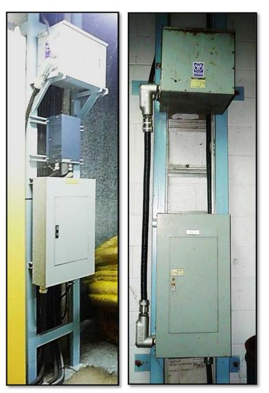
None PCB transformers atop light blue painted steel bracketry within the AREB.
