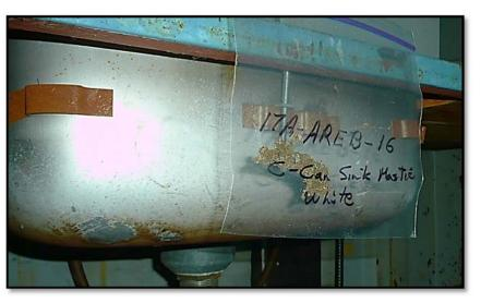
The AREB Sea-Container asbestos-containing bronze sink undercoating (sample 17A-AREB-16) painted white.
