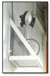
The two (2) interior emergency light fixtures mounted to the walls of the AREB have associated lead containing battery packs.
