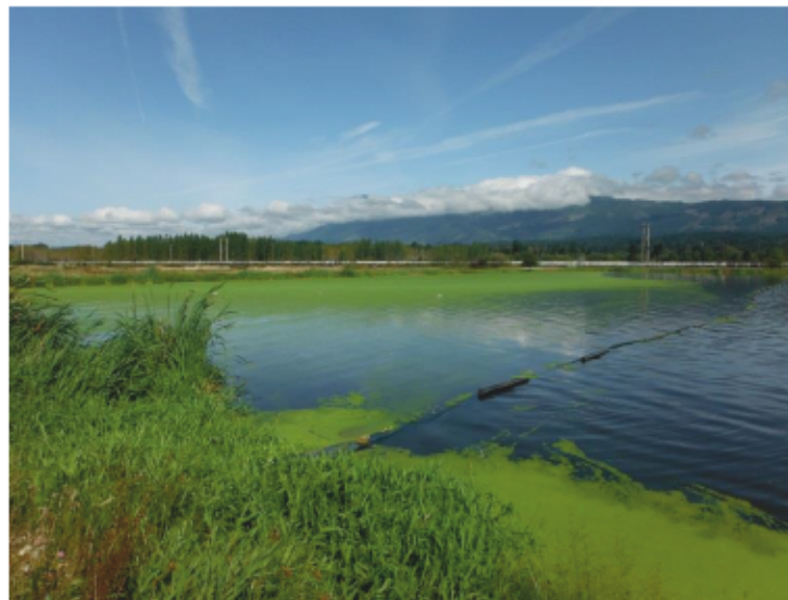
Figure 1-1 City of Port Alberni's Old Earthen Aerated Wastewater Lagoon
