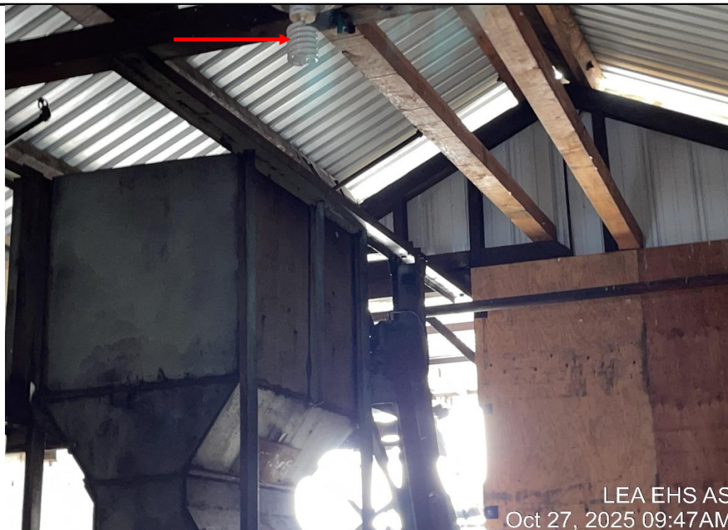
Figure 4. Mercury-Containing Compact Fluorescent Light
