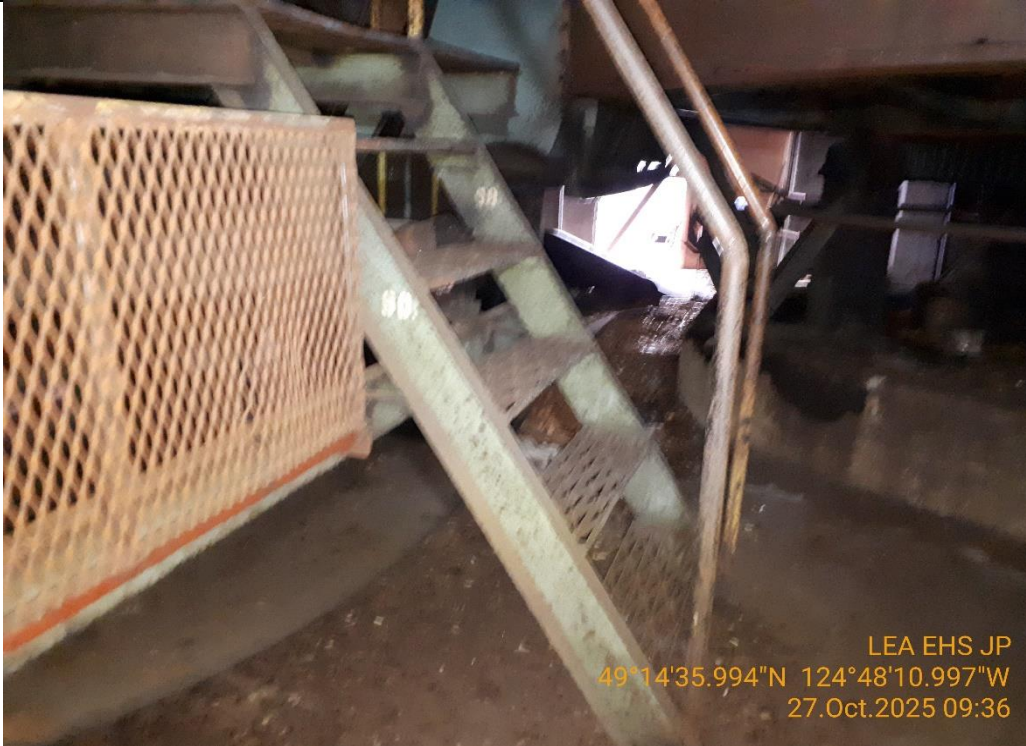
Figure 3. Lead-Containing Coatings/Metal on Interior Structures
