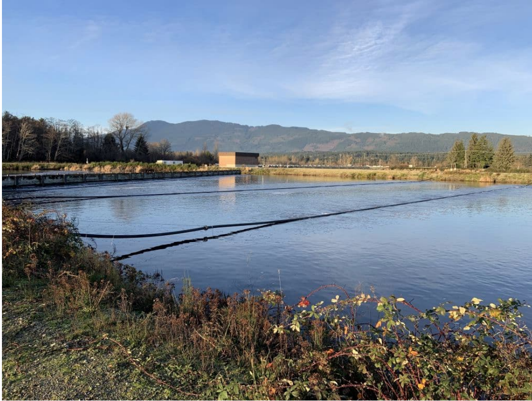
Figure 1-4 Aeration Laterals and Screening Building in Background
