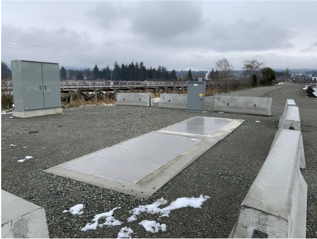
Figure 1-1 Influent Flowmeter Chambers and Sampling Kiosk
