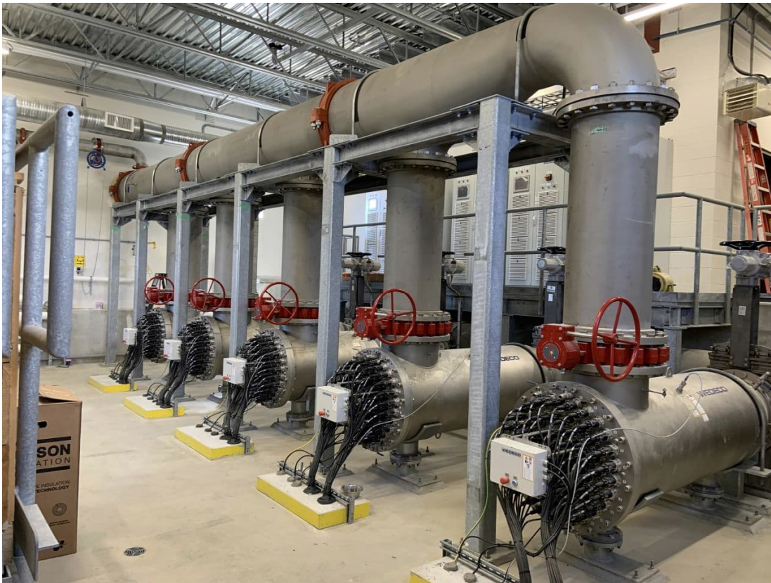
Figure 1-6 UV Disinfection
