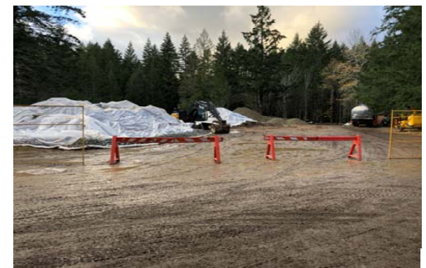
Photo 12. Soil stockpiles awaiting off site disposal.
