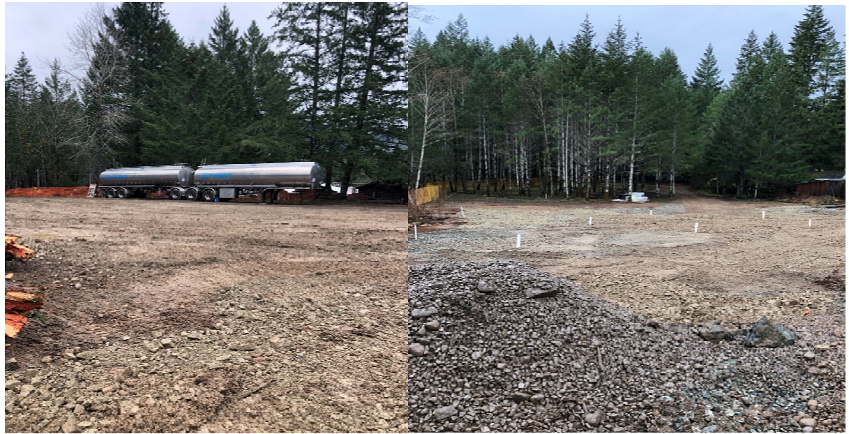
Photo 20. Tank truck filled with impacted water for offsite disposal.
