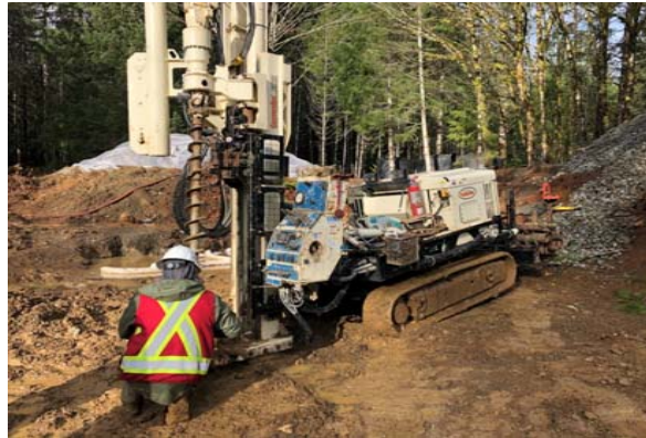
Photo 14. Soil investigation works surrounding the spill area.
