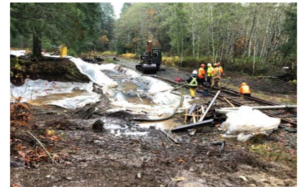
Photo 6. Initial excavation area with poly. Hydrovac cleanup of product.
