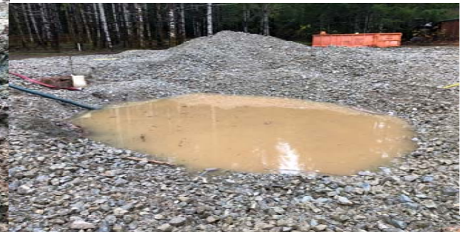
Photo 18. Backfilling excavation area and sump.
