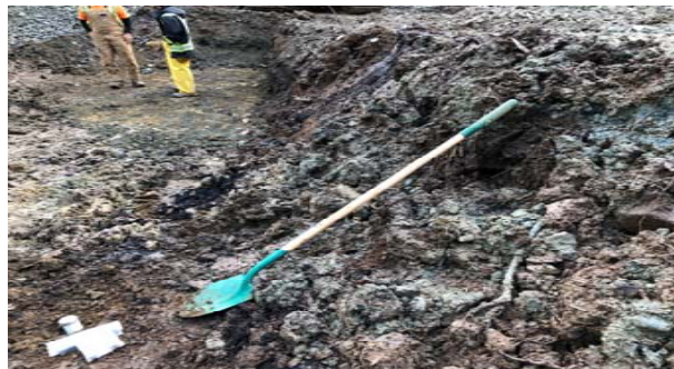
Photo 17. View of excavation works on the south wall.
