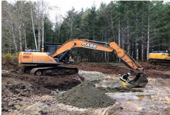
Photo 13. Track removal and soil excavation works.
