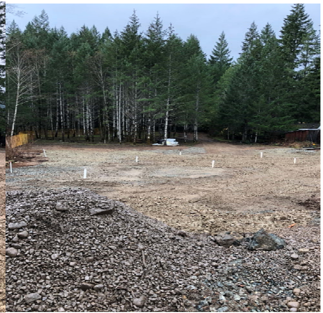
Photo 21. Final backfilling and compaction works of the excavation area.
