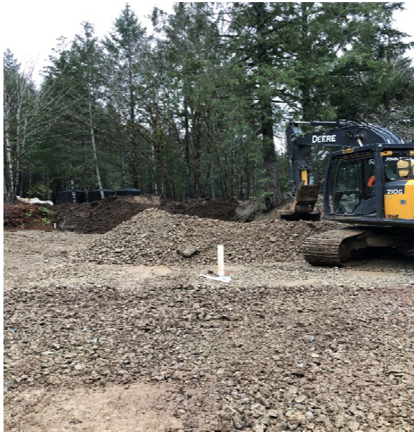
Photo 19. Installation of six recovery wells in the backfilled excavation area.
