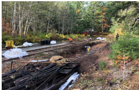
Photo 4. Initial excavation area and hydrovac cleanup.
