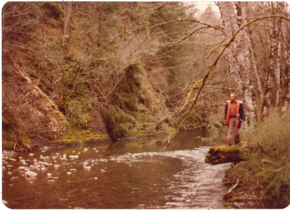
9. Crossing No. 6, 21st Avenue West looking upstream at bridge site.
