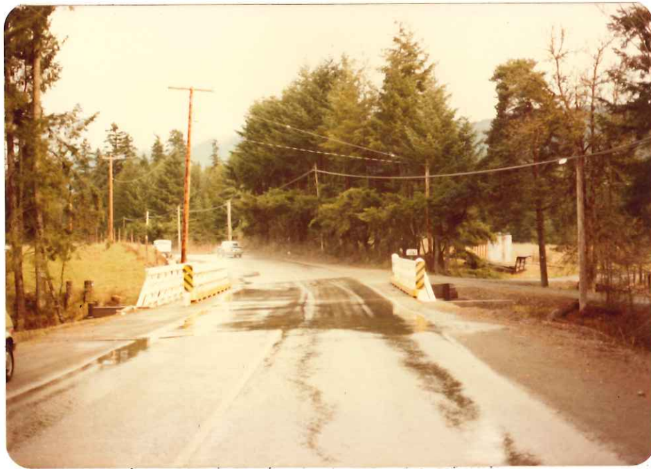
18. Cherry Creek Road Bridge.
