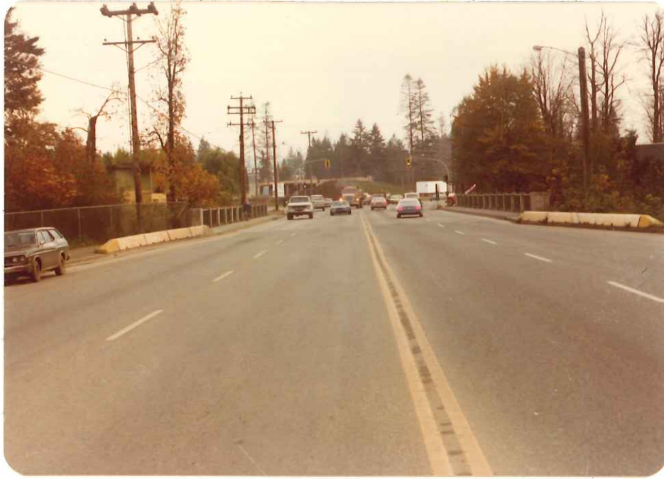
13. Gertrude Street Bridge over Rogers Creek. Looking south.
