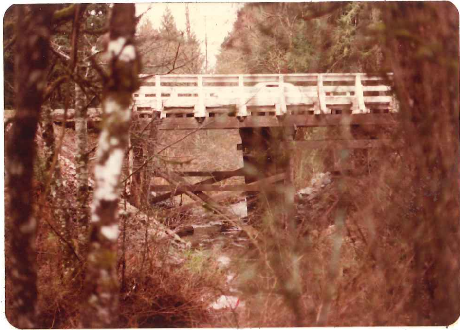
19. Cherry Creek Road Bridge looking west.
