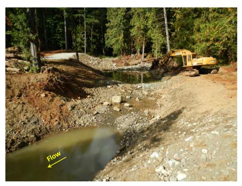
Photo 28. The channel was excavated in the "dry". However groundwater seepage filled up the pools before the creek was diverted. Spawning gravel, habitat boulders, and LWD were placed in the channel to meet the fish habitat objectives.
