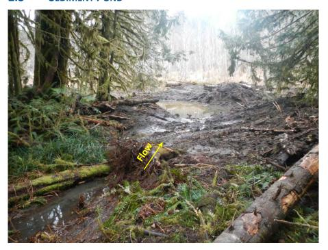
Photo 9. The sediment pond was constructed at the downstream extent of the project (Stn 2+72). Soil from the pond excavation was end-hauled to the spoil area.
