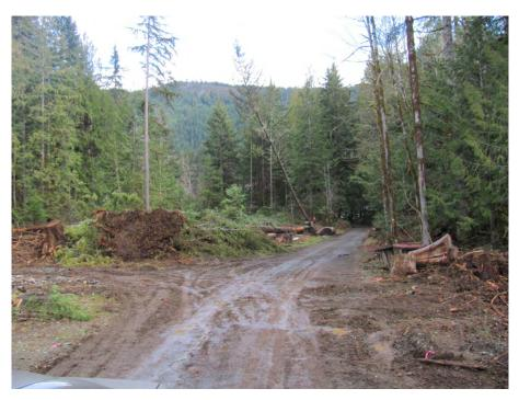
Photo 2. The new spar tree location was 75 m northeast of the bypass channel. Trees at the new setting were felled and bucked, then the stumps were removed, chipped and hauled off the site.
