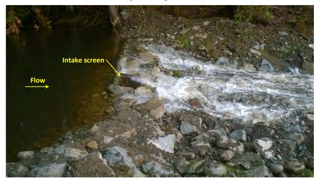
Photo 37. The intake is designed to be mainly self-cleaning, and to facilitate upstream and downstream fish passage. A fine screen keeps fish and coarse sand out of the intake.
