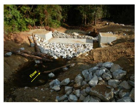
Photo 22. The fishway was backfilled with compacted till, and riprap was placed upstream and downstream of the sill. LWD and spawning gravel were placed in the channel upstream and downstream of fish fence.
