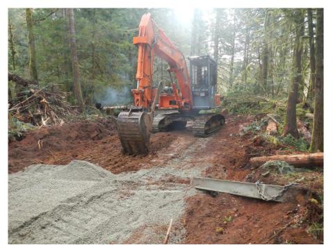
Photo 6. The glacial till was prepared by scarifying the surface, then 25 mm minus crushed rock was used to construct the saddle berm.
