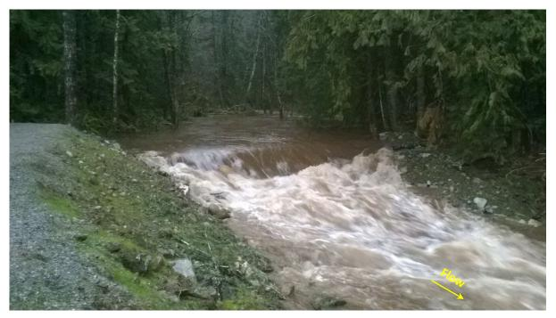
Photo 38. The December 10<sup>th</sup>, 2014 high water event was safely diverted down the new bypass channel. Flow input to the Mill Pond included direct runoff and the intake flow, the Mill Pond water level change during the flood was negligible.
