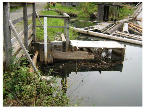
Photo 3. Fishway and Spillway with the fish counter.
