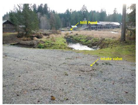
Photo 36. A 300 mm diameter steel and HDPE pipe diverts water from Kitsucksis Creek to the Mill Pond. The diversion flow is controlled by the knife gate valve housed in a concrete manhole.
