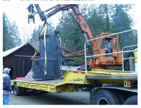
Photo 1. One of the first steps for construction was to relocate some of the heritage equipment. Here a boiler was loaded onto a lowbed using WVIIHS equipment.
