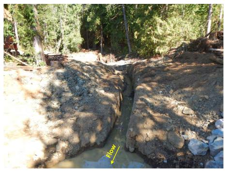
Photo 27. A drainage channel was excavated to drain the upstream area near the intake and the diversion berm.
