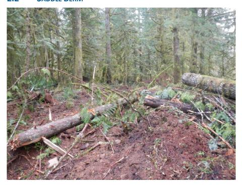
Photo 5. The saddle berm alignment was cleared and grubbed, then the topsoil was removed down to the glacial till surface.
