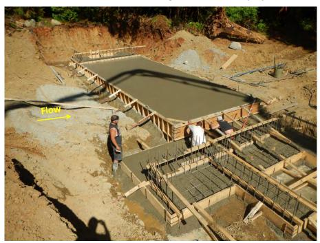
Photo 21. Concrete was poured and finished by Athecon Projects Inc. The concrete cured for a week before it was stripped and backfilled.
