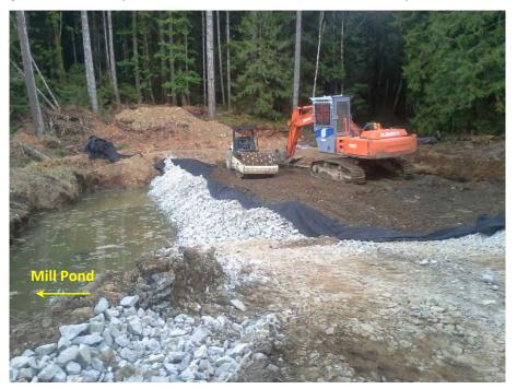
Photo 33. The saddle berm was mainly constructed with compacted till excavated from the new bypass channel.
