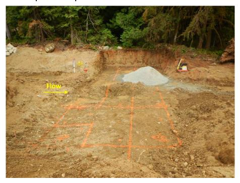
Photo 19. The fish fence was layed out on the ground with marker paint and then a small excavator was used to grade the surface.
