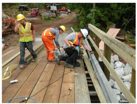
Photo 15. The bridge was widened, sandblasted, and painted. Then City of Port Alberni staff installed the decking, guard rails, and hand rails.
