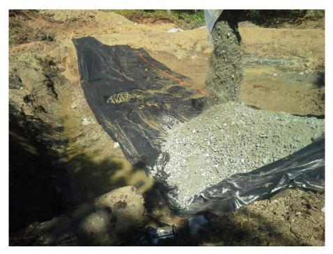
Photo 32. Overburden at the diversion berm area end-hauled to the spoil area. The underlying glacial till was exposed and a rock filter was constructed as part of the structure.
