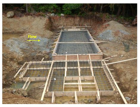
Photo 20. The formwork and reinforcing were installed in preparation for the concrete pour.
