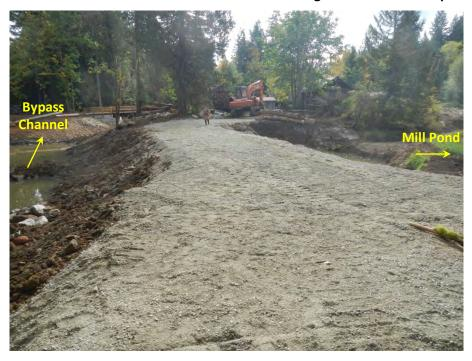
Photo 35. The riprap was keyed into the channel bed and placed up the creek-side slope. The riprap was covered with gravel and vegetated with grass seed.
