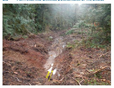
Photo 17. The channel was cleared and grubbed, the photo shows the alignment from Stn 1+30 to 1+70.
