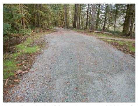
Photo 8. The completed saddle berm surface was crowned slightly to reduce rainfall pooling, and the side areas were smoothed out and vegetated with grass seed.
