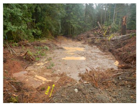
Photo 18. The topsoil was stripped down to the glacial till. The excavated material was end-hauled and stockpiled in the spoil area.
