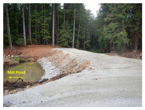
Photo 34. The completed diversion berm had the banks graded at 2:1 slope and the surface covered with 25 mm minus crushed rock with a slight crown to reduce pooling of rain water.
