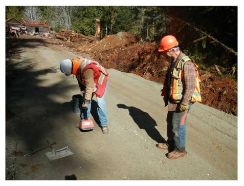
Photo 7. The saddle berm was compacted with a vibratory roller compactor, and then a nuclear densometer was used to test the compaction levels.
