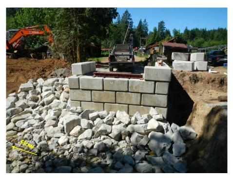
Photo 14. Riprap was placed around the abutment to protect them from scour.
