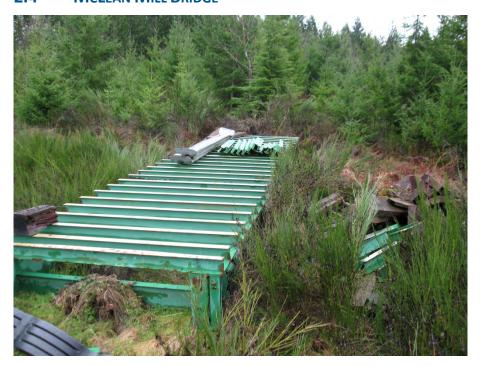
Photo 11. BC Timber Sales donated a steel bridge that was refurbished and installed over the bypass channel.
