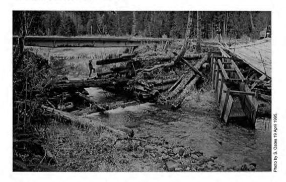
View looking upstream of breach in millpond dam on Kitsuksis creek. The fish ladder in the right portion of the photo will be removed and replaced with a combination spillway and fish ladder.
