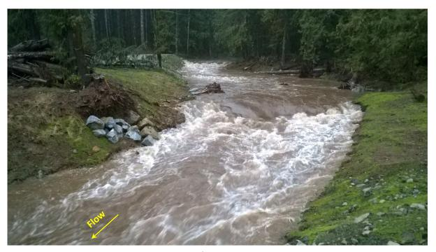
Photo 30. A significant flood on December 10<sup>th</sup>, 2014 caused some minor bank erosion immediately upstream of the bridge near Stn 0+70, but the channel held up well overall.
