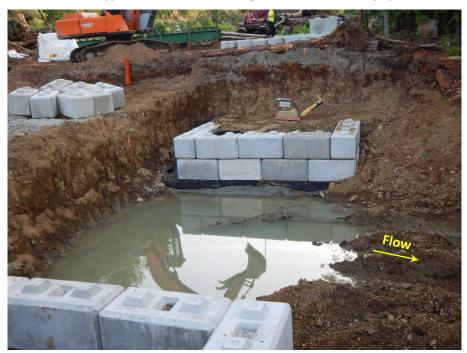
Photo 13. The channel was excavated to the subgrade and the bridge abutments were set using crushed rock, geo-grid, and lock blocks.
