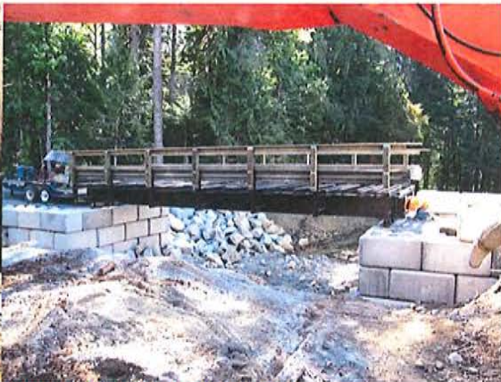
View of the new stream channel
