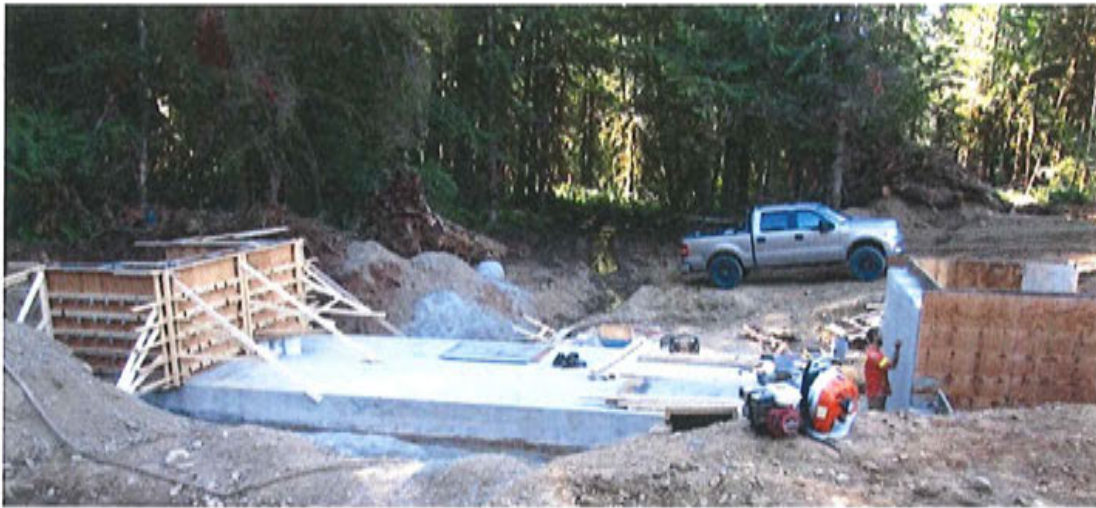
Fish Fence foundation, July 2014.
