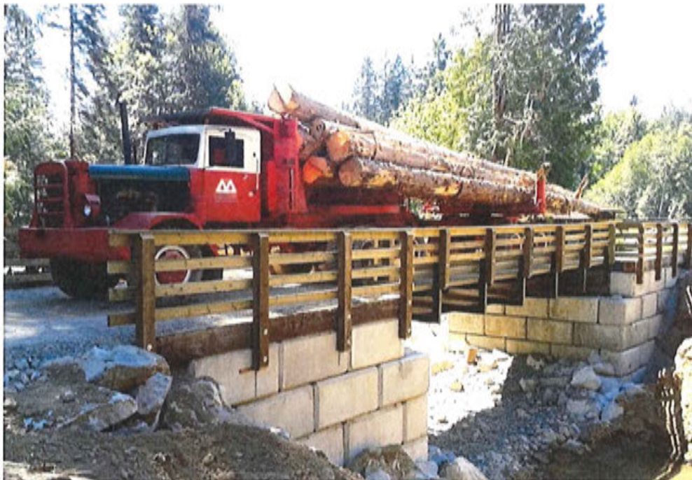
First load over the completed bridge – July 15, 2014.
