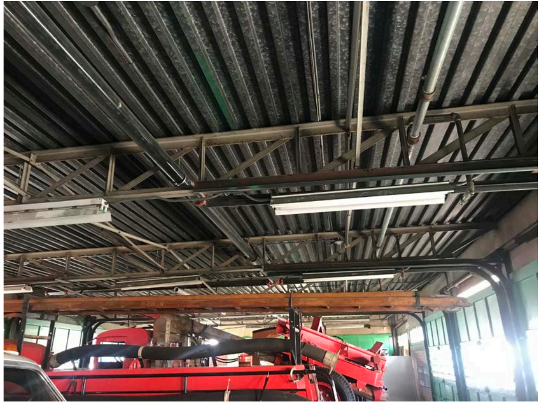
The truck garage is a simple steel and concrete structure with uninsulated walls and roof
