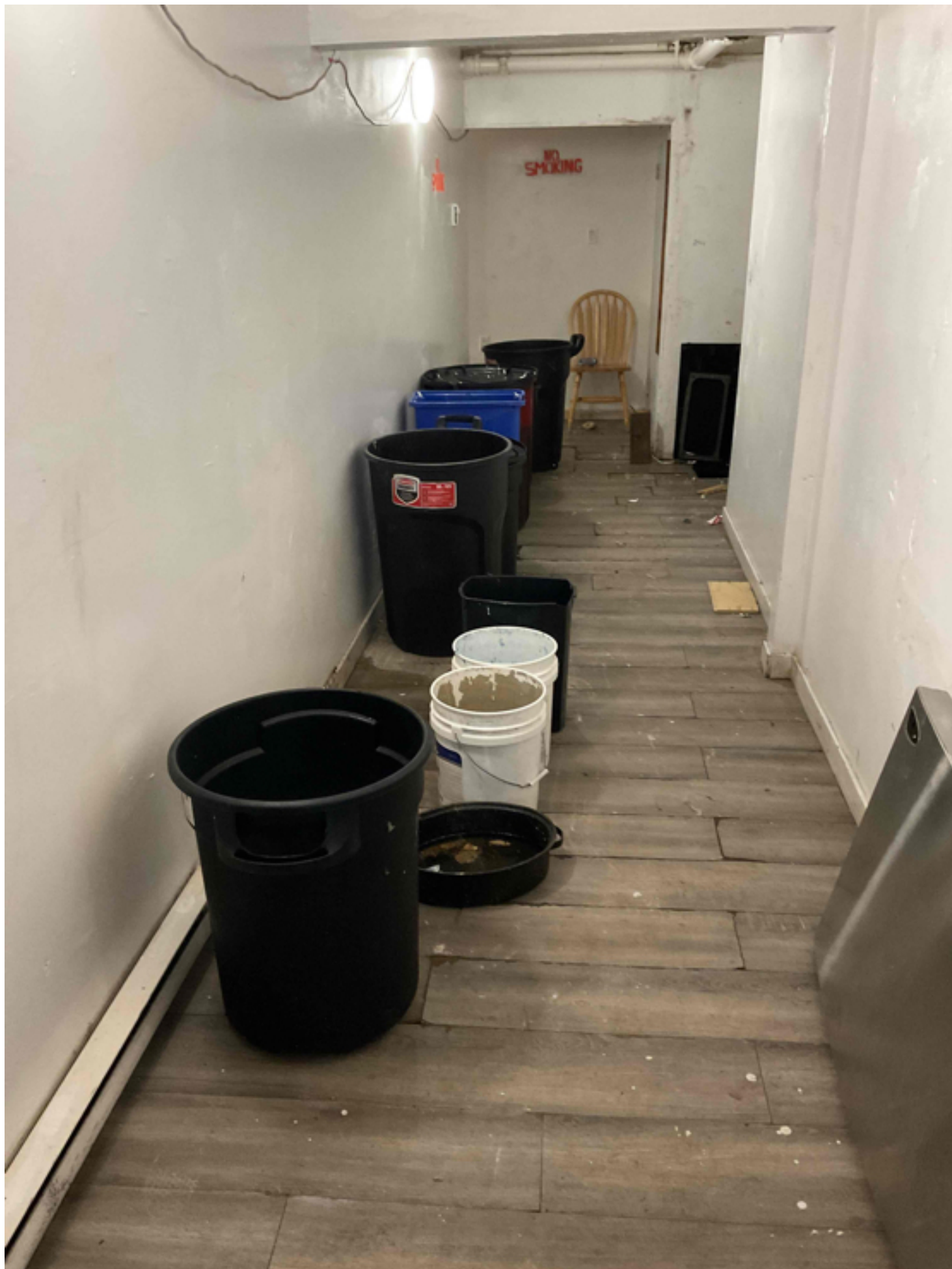
3rd floor east end- combustible containers blocking path to exit.
