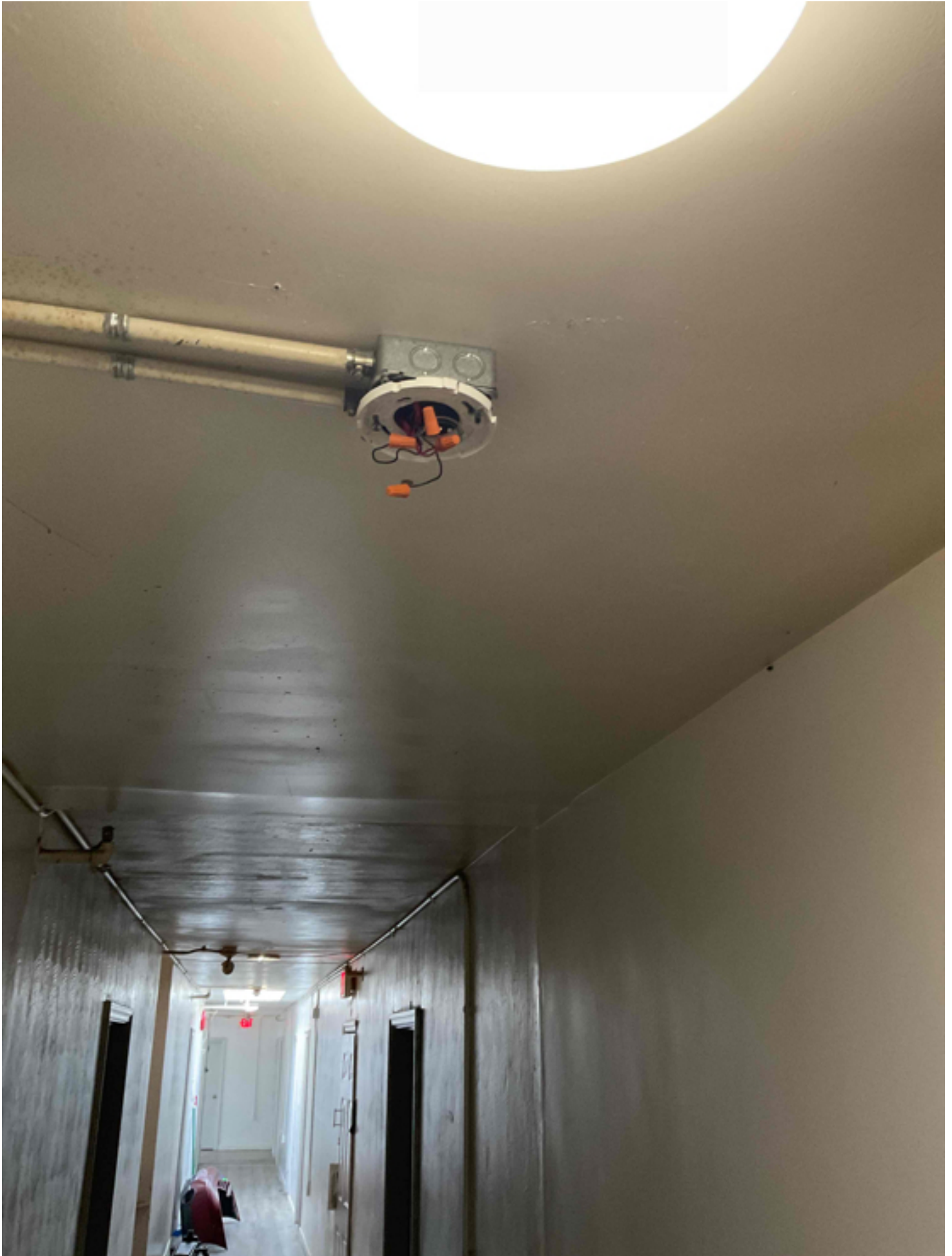
3rd floor missing detector
