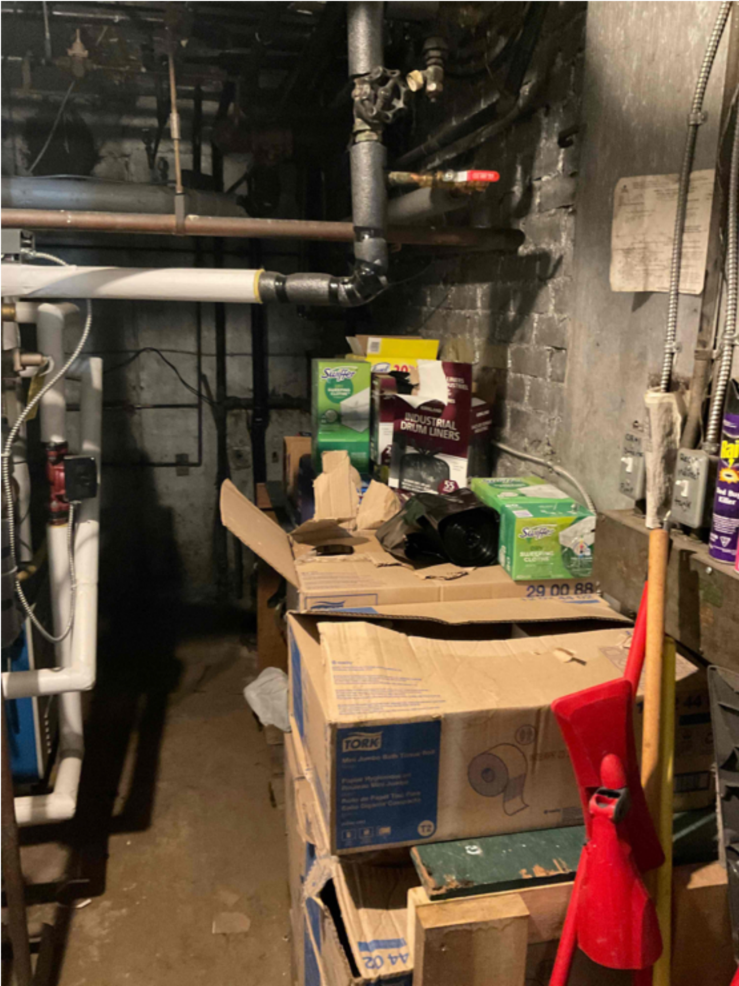
boiler room - combustible storage
