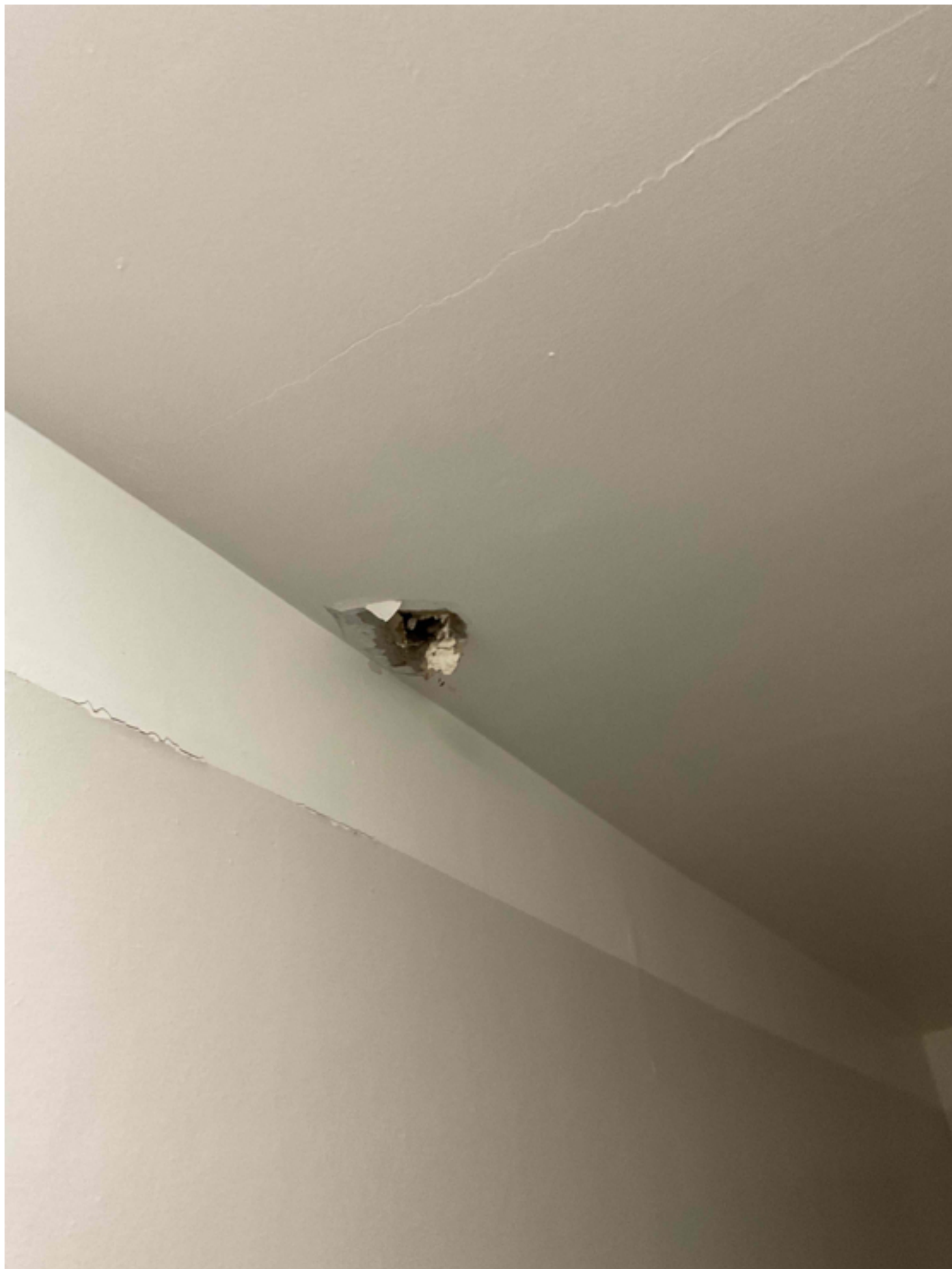
2nd floor ceiling drywall seperation
