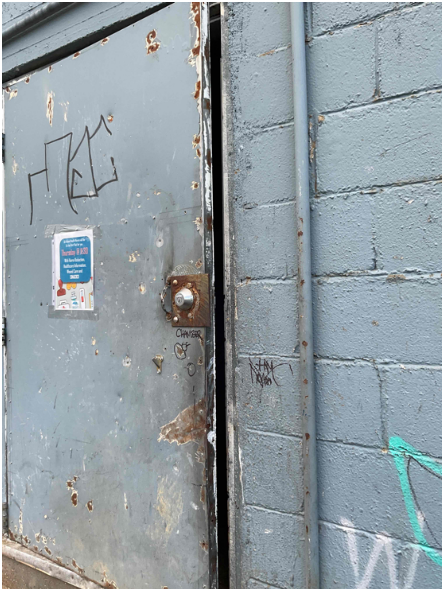
3rd floor, east end emergency exit doesn't close and latch
