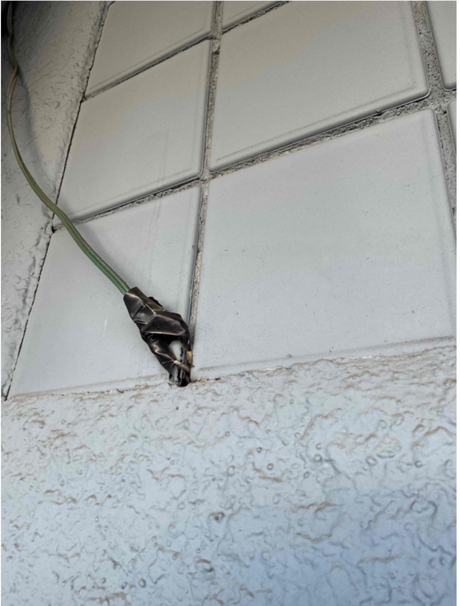
improper wiring on signs at pub entrance
