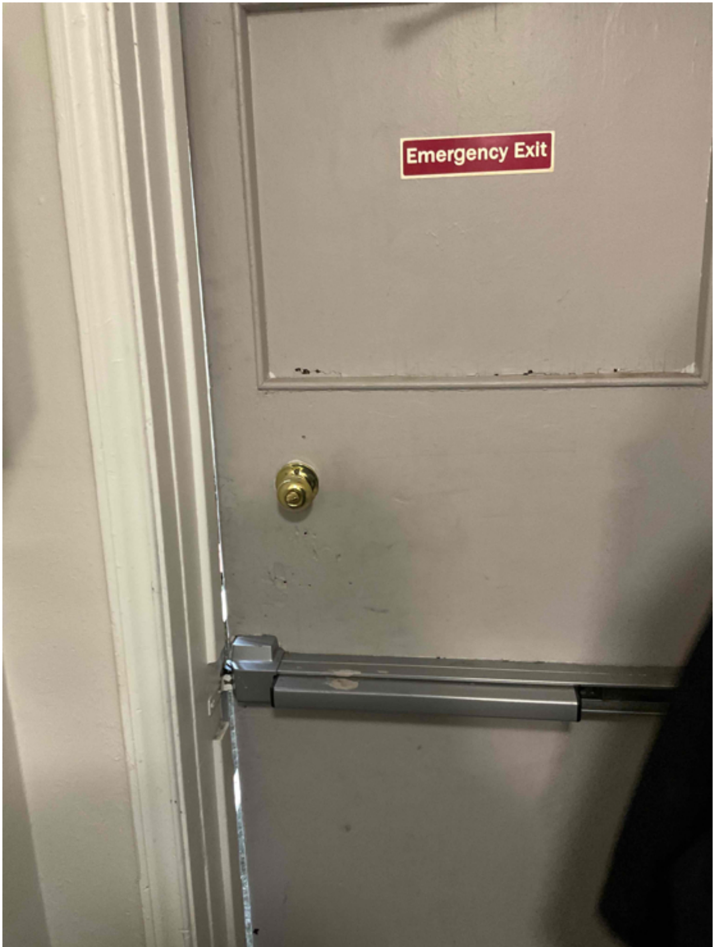
2nd floor fire escape door doesnt close and latch
