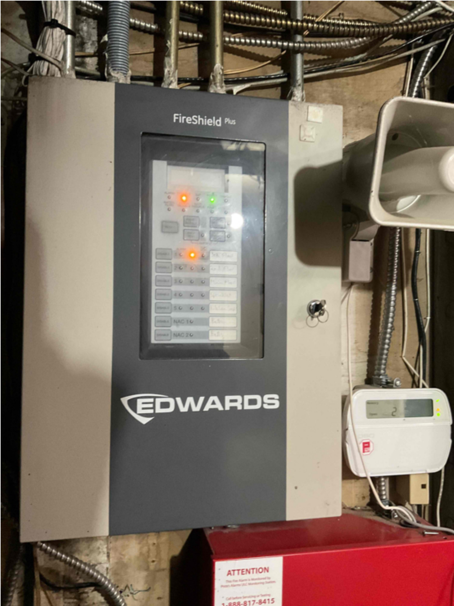
fire alarm still in trouble mode
