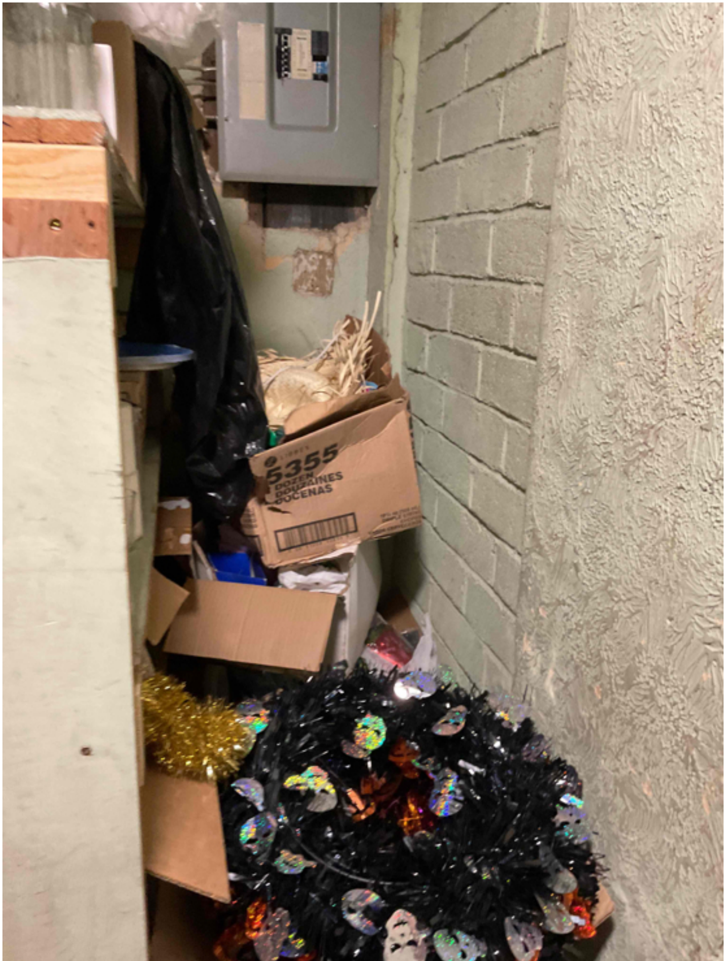
combustible storage in front of electrical panel - downstairs.
