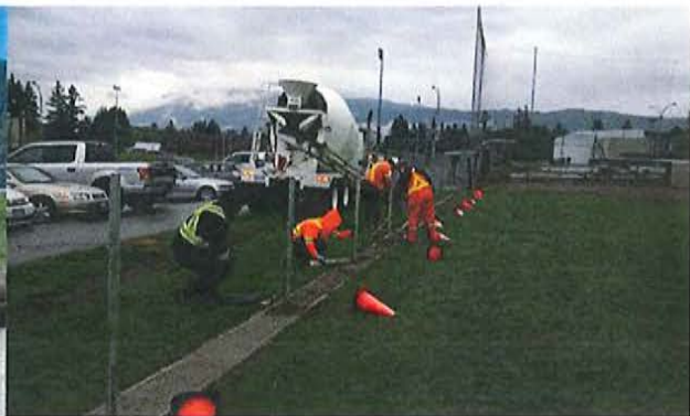
Fence installation – Preparing for seasonal play
