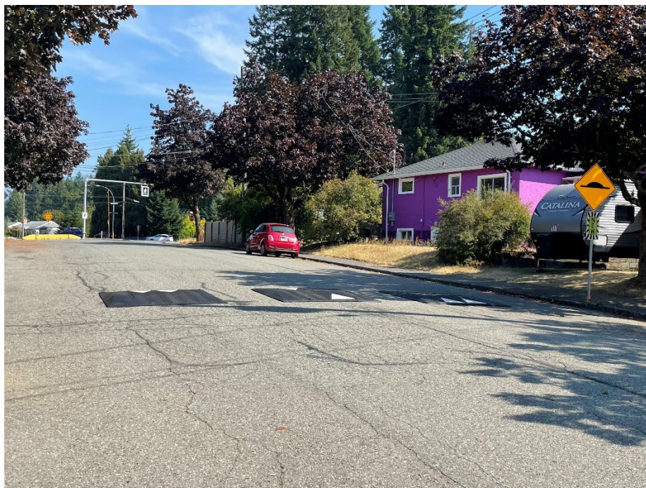
Figure 7: New Speed Cushions Installed on Princess Street
