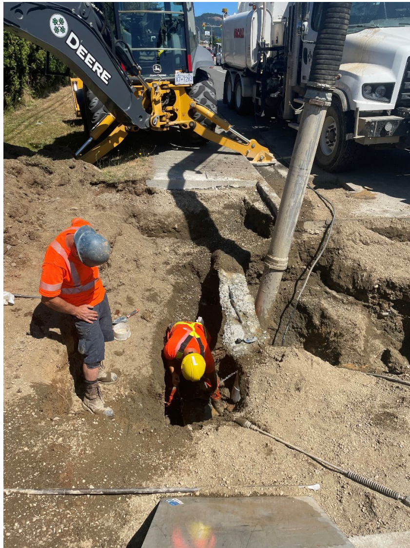
Fig 5: Watermain Repair on Johnston Road
