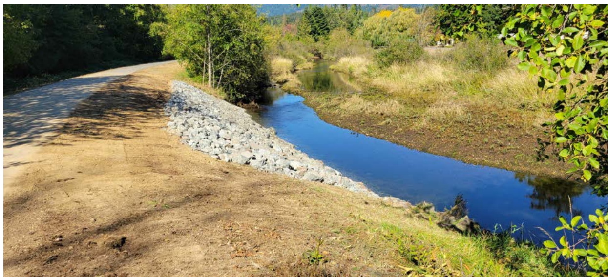
Fig 4: Kitsuksis Dike West Embankment Rehabilitation
