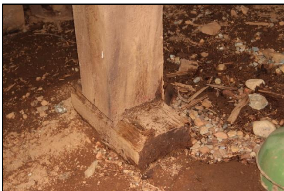
Photographs 125 - 128 – (clockwise from top left) renewed timber deck structure, organic growth on original timber beam, deteriorating post base, , deteriorating timber footing
