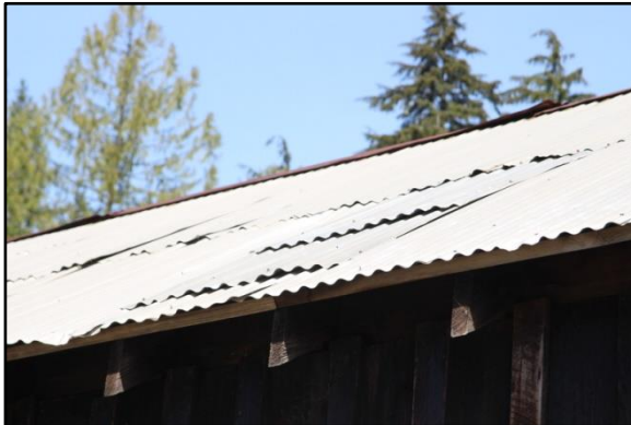
Photographs 75 - 77 – (clockwise from top left) loose corrugated roof sheet, deteriorating cladding at base of wall, untrimmed window opening
