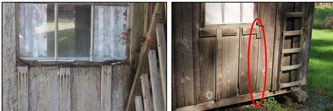
Photographs 41 - 42 – (left to right) missing window trim and debris accumulation at the base, missing batten
