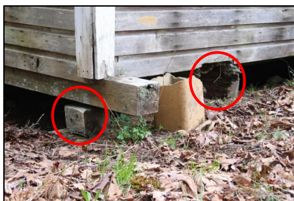
Photographs 44 - 46 – (clockwise from top left) lifting and buckling sheet metal roof, settled and deteriorating timber footing assembly
