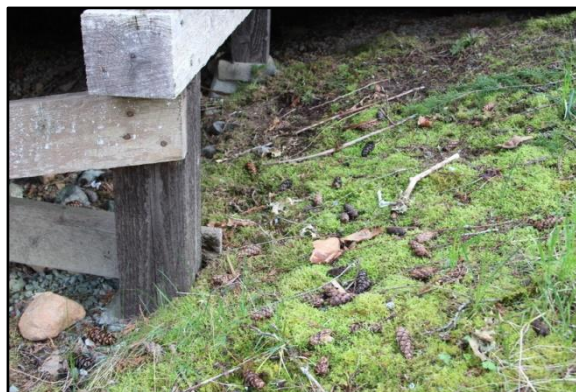
Photograph 27 –grade encroaching on a foundation post.
