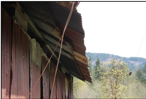
Photographs 92 - 94 – (clockwise from top left) Double layer roof assembly over the east building, gaps between the roof cladding and chimney, sheet rubber lined, wood frame gutters
