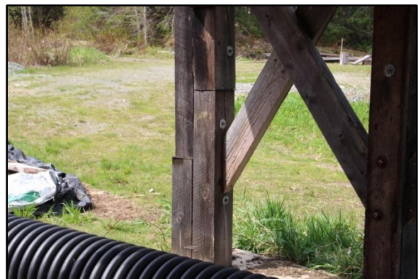
Photographs 130 - 132 – (clockwise from top left) Corroded, corrugated metal roof with flipped panel, spliced posts supporting the Waste Sheds
