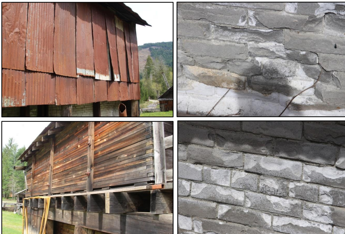
Photographs 95 - 98 – (clockwise from top left) corroding sheet metal wall cladding, spalling and eroding brick foundation, laminated timber walls
