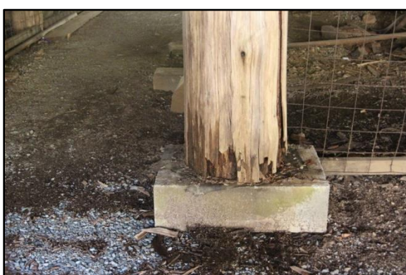
Photographs 125 - 128 – (clockwise from top left) renewed timber deck structure, organic growth on original timber beam, deteriorating post base, , deteriorating timber footing
