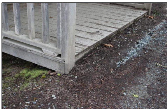
Photograph 25 & 26 – (left to right) grade accumulation along the north elevation
