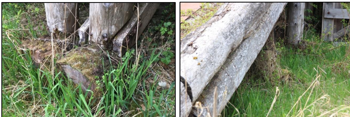
Photographs 108 & 109 – (left to right) timber footings set on grade being overgrown and deteriorating
