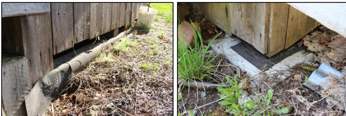
Photographs 89 & 90 – (left to right) protective sheet rubber between the timber structure and concrete footings
