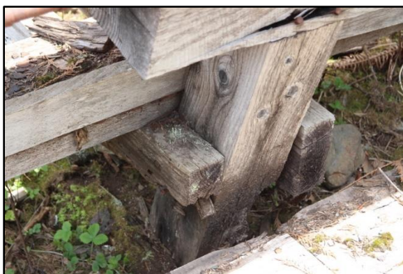
Photographs 122 & 123 – (left to right) failed timber joints
