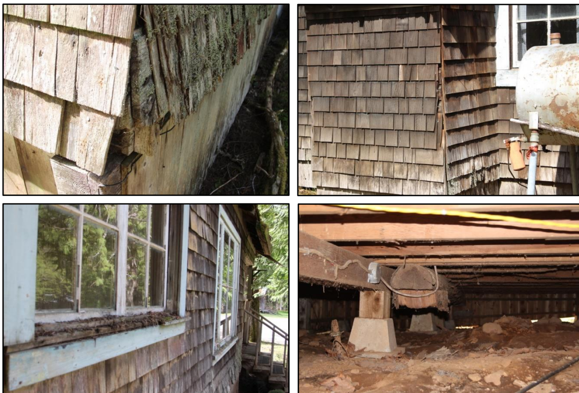
Photographs 13 - 16 – (clockwise from top left) deteriorated wall cladding, sound building frame and footings, debris on the window sills
