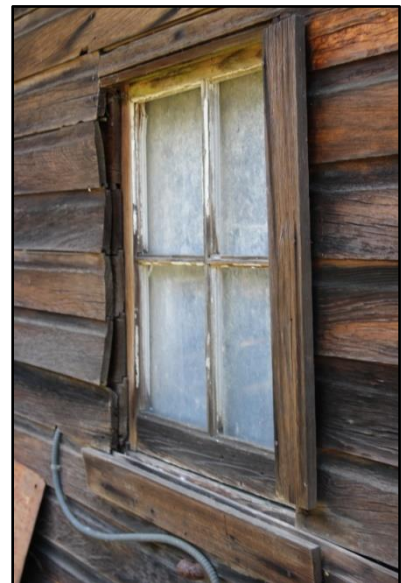
Photographs 149 - 151 – (clockwise from top left) buckled corrugated roof panel, damaged wall siding, missing trim on the north window
