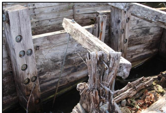
Photographs 146 & 147 – (left to right) structural deterioration of the planks and timbers
