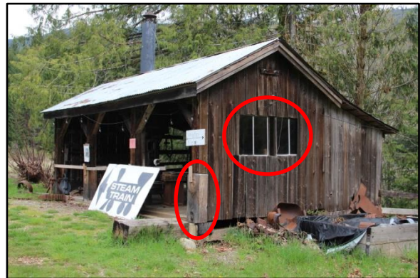
Photographs 87 & 88 – (left to right) organic debris accumulation on the sheet metal roof, unsympathetic post repair and sliding sash
