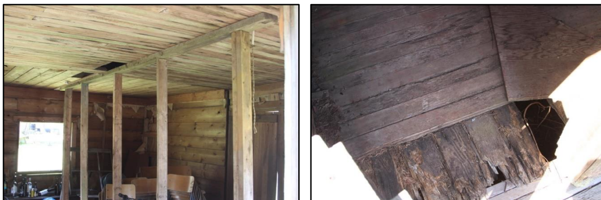
Photographs 51 & 52 – (left to right) interior stud wall, overlaid, deteriorating floor planks
