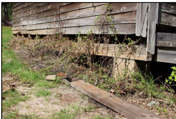
Photographs 48 - 50 – (clockwise from top right) deteriorated timber roof structure, north porch with adjacent door and cladding deterioration, perimeter growth
