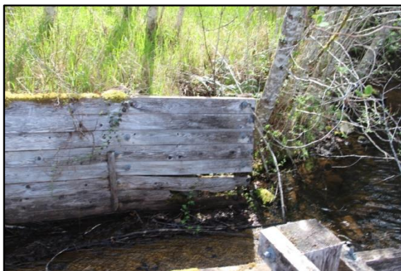
Photographs 146 & 147 – (left to right) structural deterioration of the planks and timbers
