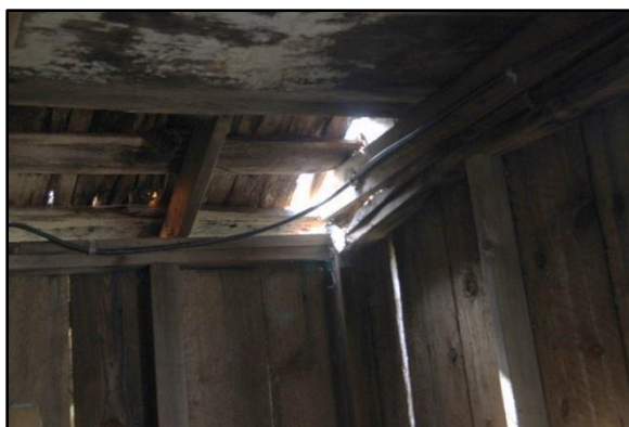
Photograph 18 - 20 – (clockwise from top left) damaged roof tarp, holes through the main, cedar shingle roof and the lean-to, sheet metal roof
