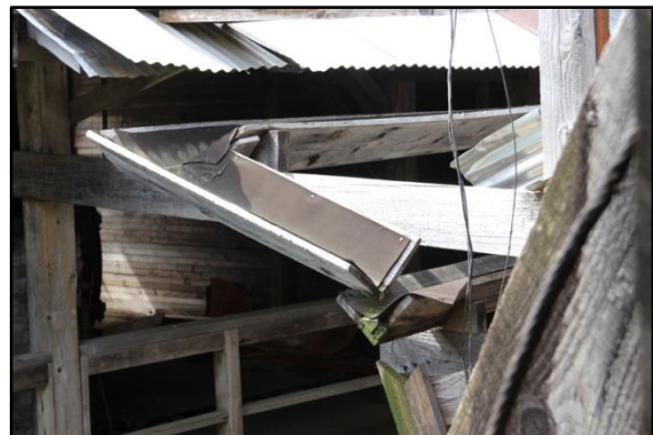
Photographs 92 - 94 – (clockwise from top left) Double layer roof assembly over the east building, gaps between the roof cladding and chimney, sheet rubber lined, wood frame gutters
