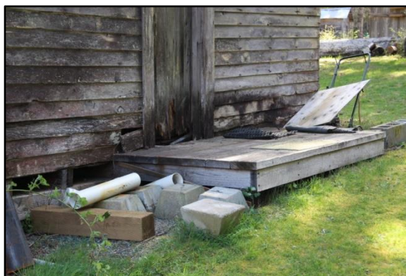
Photographs 48 - 50 – (clockwise from top right) deteriorated timber roof structure, north porch with adjacent door and cladding deterioration, perimeter growth
