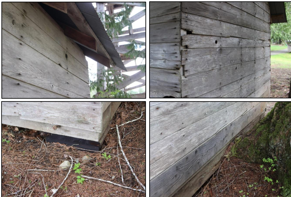
Photographs 33 - 36 – (clockwise from top left) sheet metal roof cladding overhang, deteriorated siding, building base constructed over a tree root, a creosote block footing
