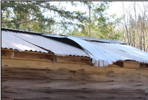
Photographs 149 - 151 – (clockwise from top left) buckled corrugated roof panel, damaged wall siding, missing trim on the north window
