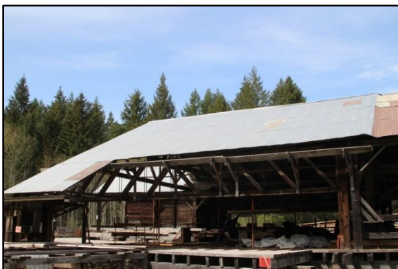
Photographs 111 & 112 – (left to right) renewed west roof, double roof over the planer
