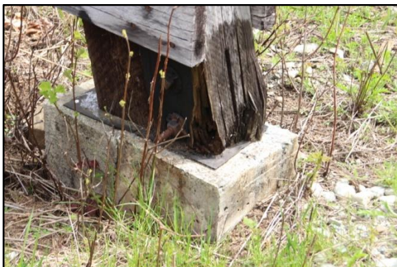
Photographs 133 - 135 – (clockwise from top left) treated and deteriorated timber post base of a Conveyor Belt frame, corroded steel frame, corroded and dilapidated Burn Pile structure
