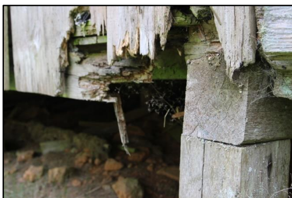
Photographs 8 - 10 – (clockwise from top left) renewed timber foundation structure on concrete pad footings, deteriorated exterior joists resulting in building displacement
