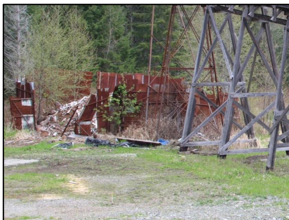
Photographs 133 - 135 – (clockwise from top left) treated and deteriorated timber post base of a Conveyor Belt frame, corroded steel frame, corroded and dilapidated Burn Pile structure
