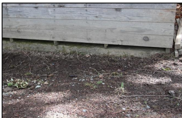
Photograph 25 & 26 – (left to right) grade accumulation along the north elevation
