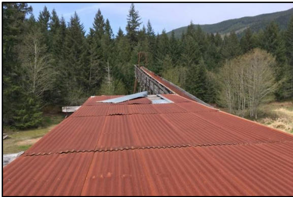
Photographs 130 - 132 – (clockwise from top left) Corroded, corrugated metal roof with flipped panel, spliced posts supporting the Waste Sheds
