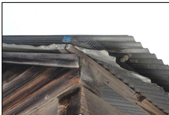
Photographs 111 & 112 – (left to right) renewed west roof, double roof over the planer
