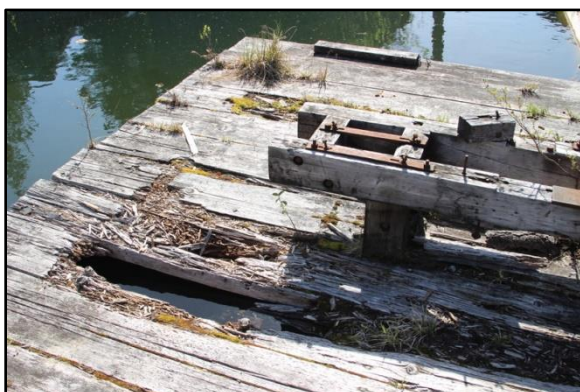
Photographs 84 & 85 – (left to right) Deteriorating wood planks, corroding piece of mechanical equipment
