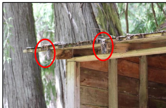
Photograph 24 – debris runoff on the rafter tails
