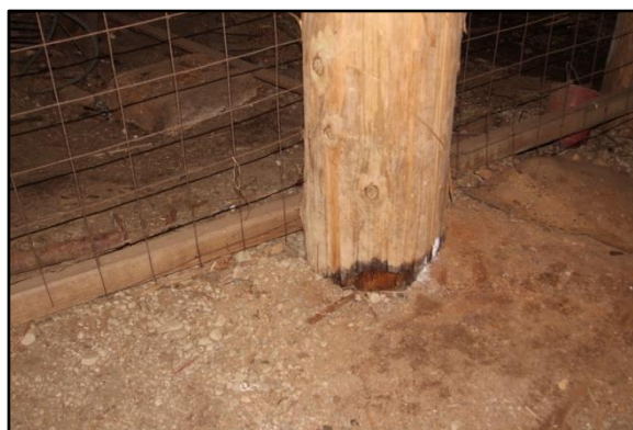
Photographs 118 & 119 – (top to bottom) repaired wall post, deteriorating foundation post base
