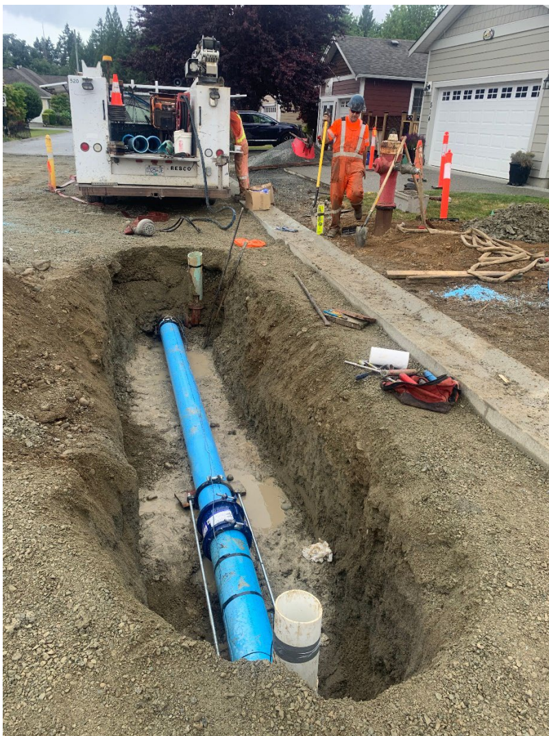
Figure 1: New Water Main Extension & Installation on Pierce Road
