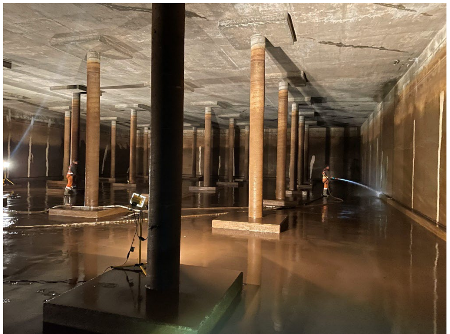
Figure 2 – Johnston Reservoir cleaning
