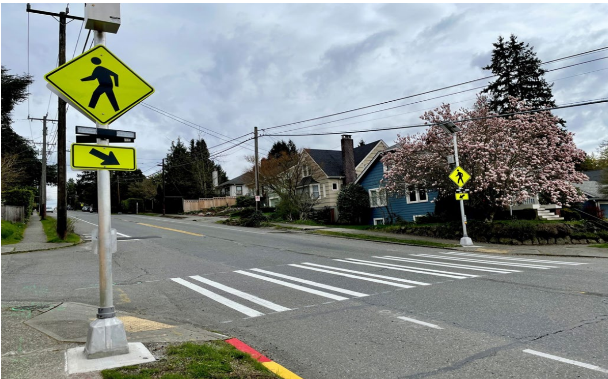
Figure 1: Typical RRFB Installation at Crosswalk
