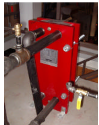
Figure 6 District Energy Heat Exchanger
