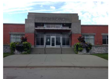
Cleaning the exterior of the RCMP detachment
