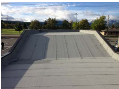
Echo Centre Canopy roof replacement
