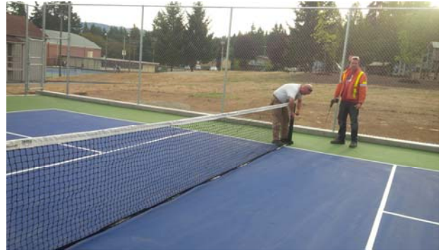
Pickle ball court - perimeter drains and landscaping still to be completed.
